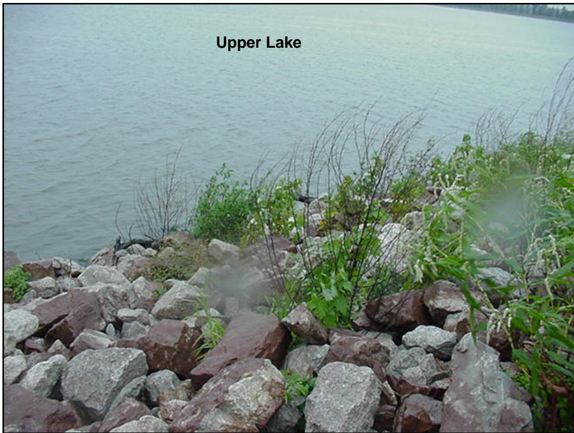
Photograph C-5 .Northern perimeter levee riprap protection placed by USFWS. (August 2004)
