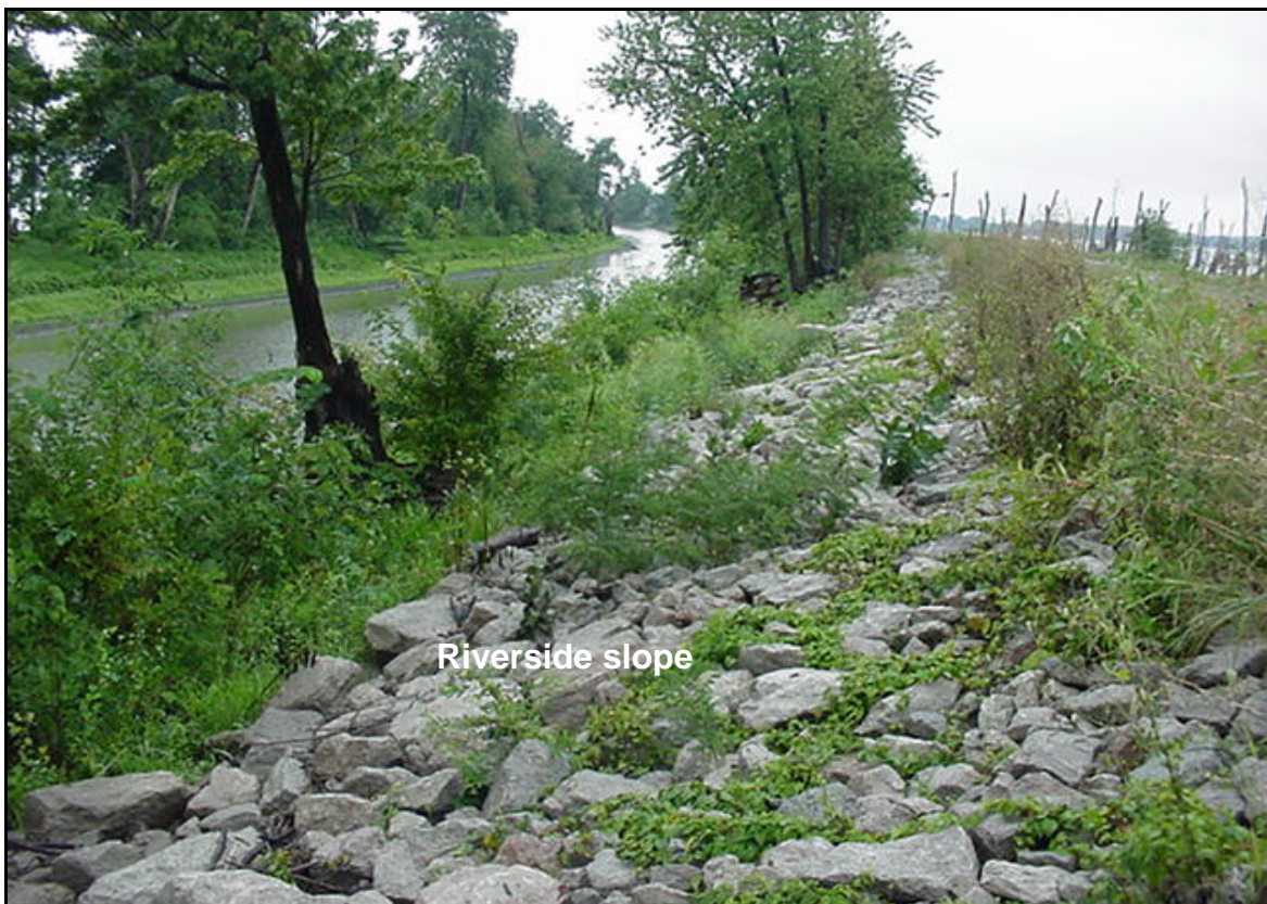
Photograph C-4. Northern perimeter levee riprap protection placed by USFWS (August 2004)
