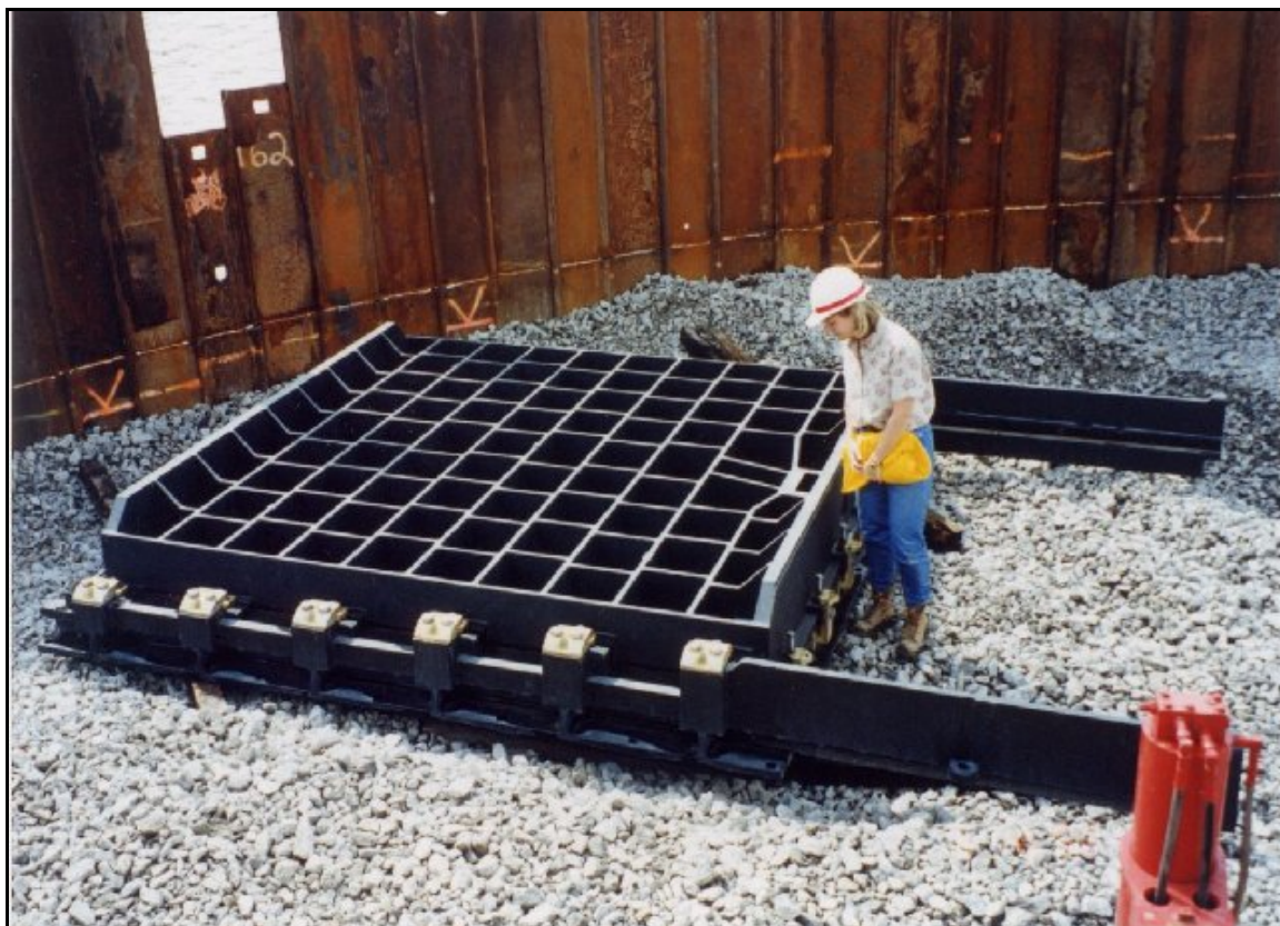
Photograph C-8. Sluice Gate (During Construction)
