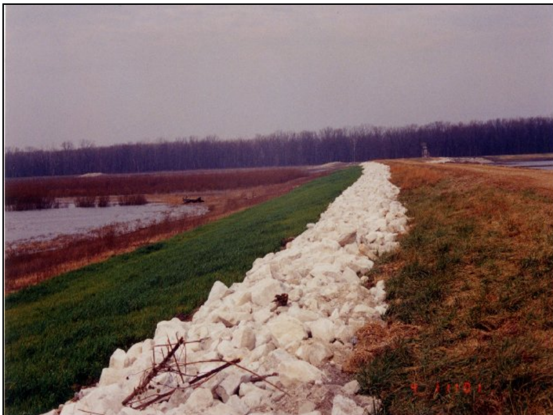
Photograph C-2. Completed Cross Dike Levee with Riprap Protection
