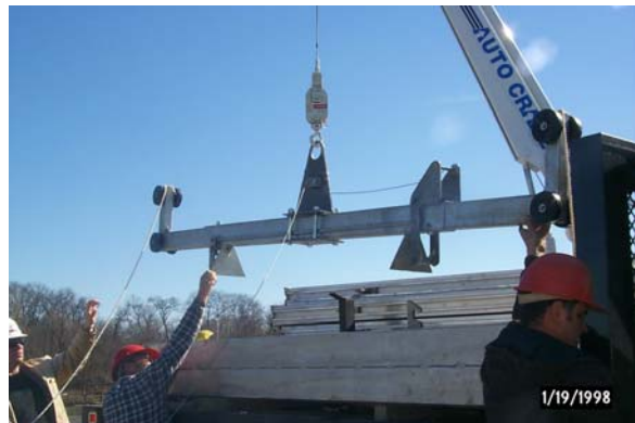
34. Lake Chautauqua. Lifting beam for 10 ft wide aluminum stoplogs.
