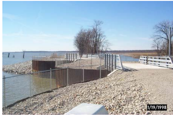
33. Lake Chautauqua. Cellular Water Control Structure.
