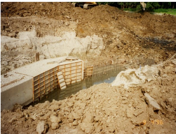
13. 5x5 Box Culvert from pump station to the river under construction.
