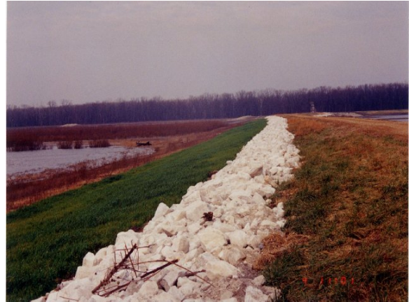
9. Cross Dike levee looking toward the river. Lower Lake side has a 6:1 slope. Band of riprap protects against wave wash erosion at higher river levels.
