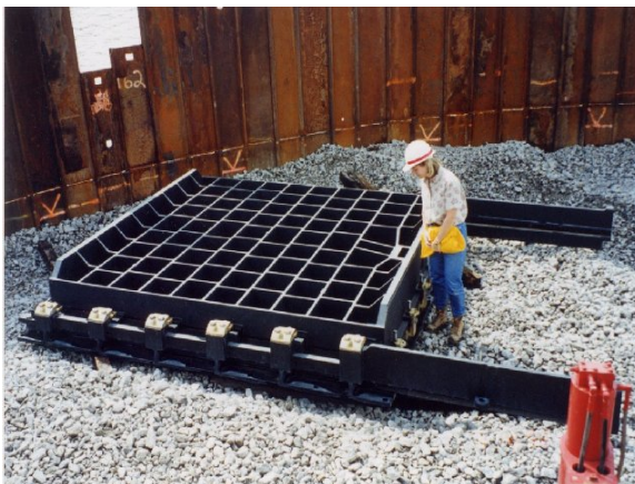
3. 10ft by 10ft Sluice Gate prior to installation. 74ft diameter sheet pile cell is filled with rock.
