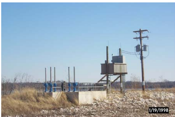
26. Lake Chautauqua. 41,000 GPM pump station and electrical control platform/transformers.
