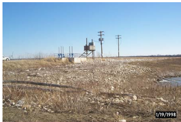
27. Lake Chautauqua. 41,000 GPM pump station and electrical control platform/transformers. Lower Lake outlet is shown.
