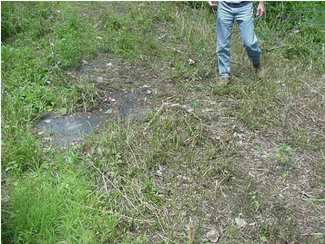
Photo 6. Exposed Fabric on Causeway
