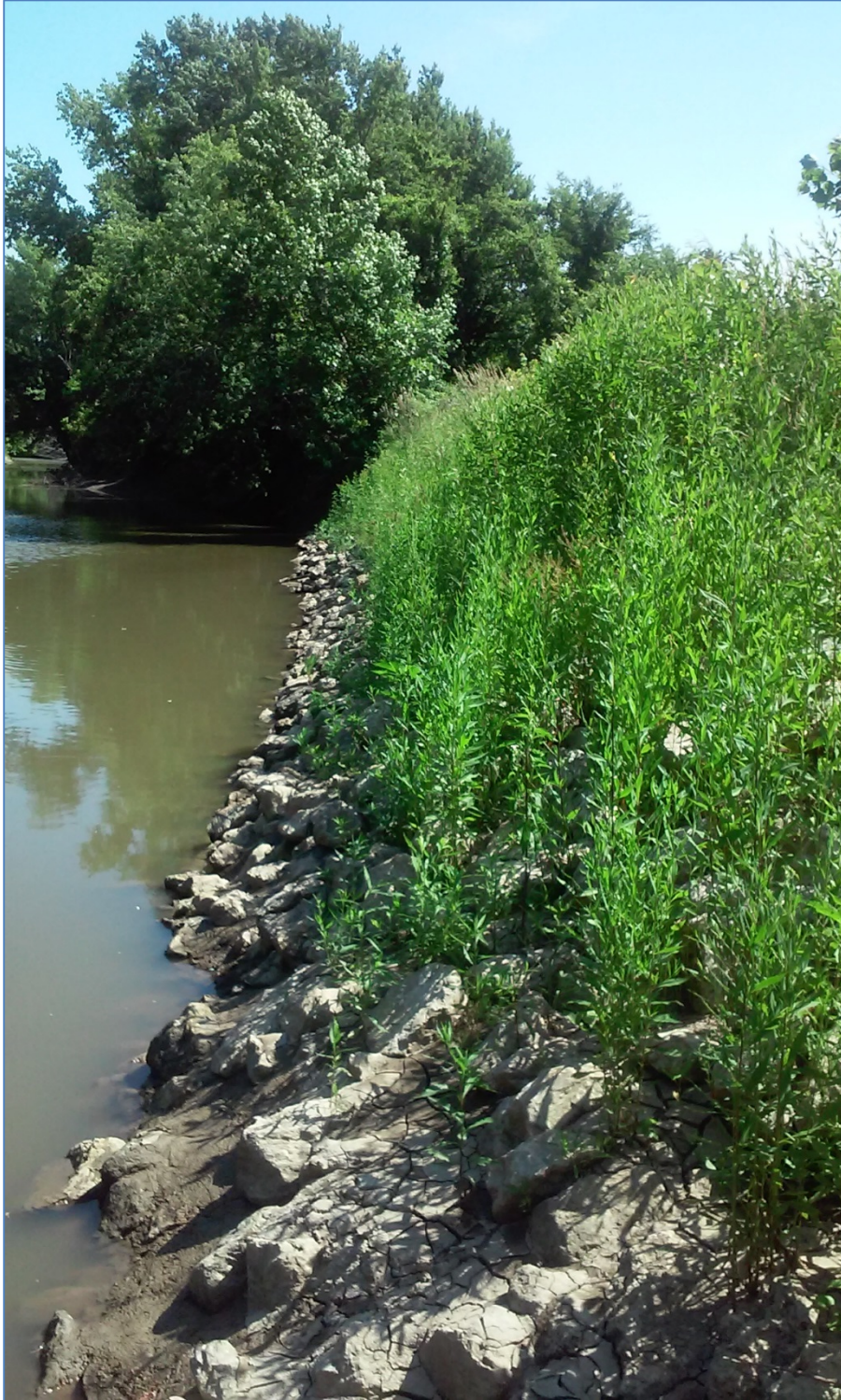
Photo #10 – Riprap upstream of Stoplog C. Moderate vegetation in riprap.
