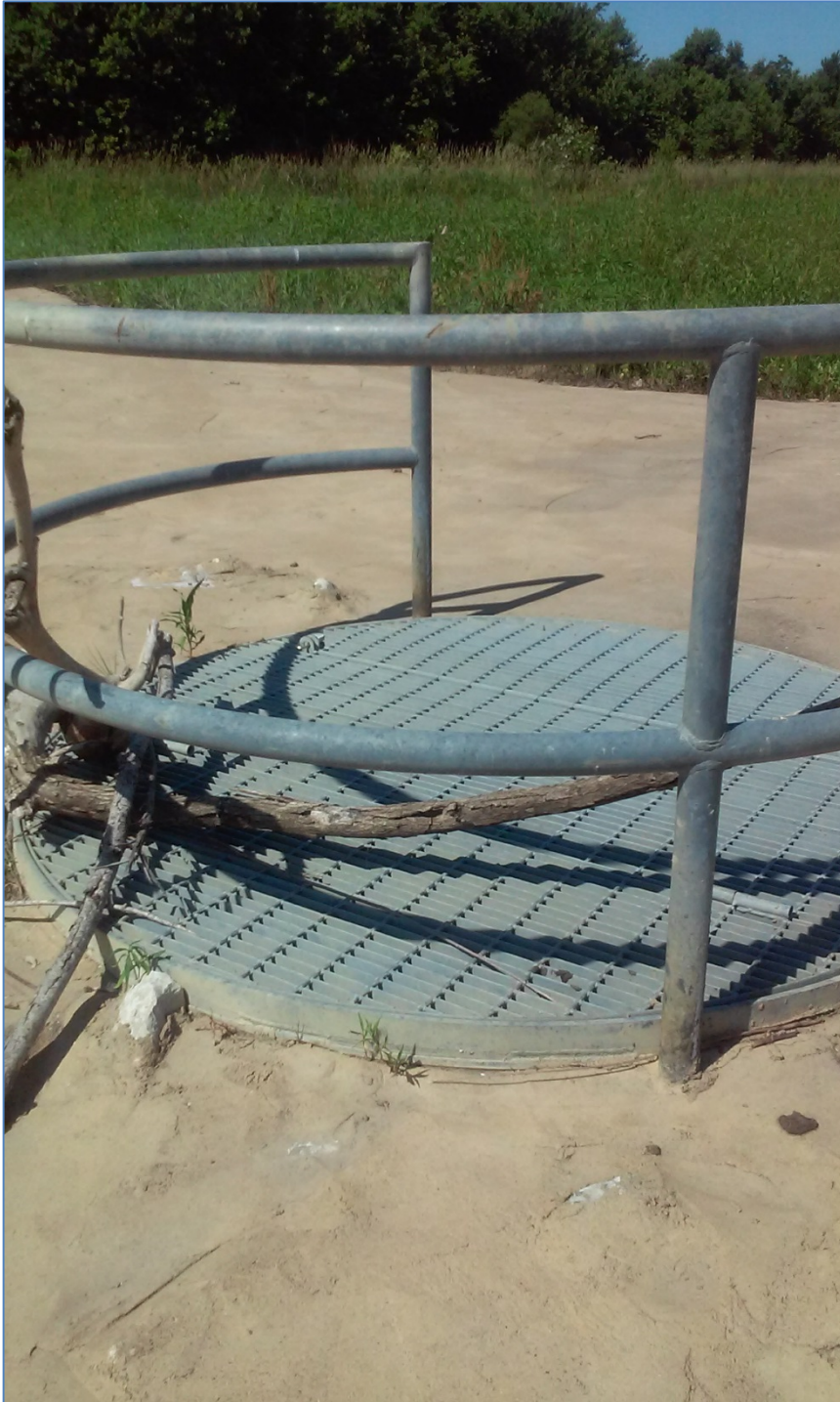
Photo #15 – Stoplog D, debris in railing.
