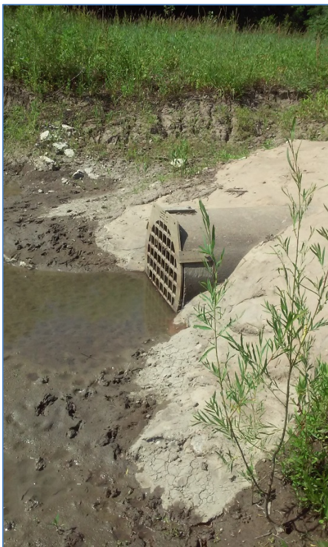
Photo #13-Stoplog D, upstream gate, bank erosion in background.
