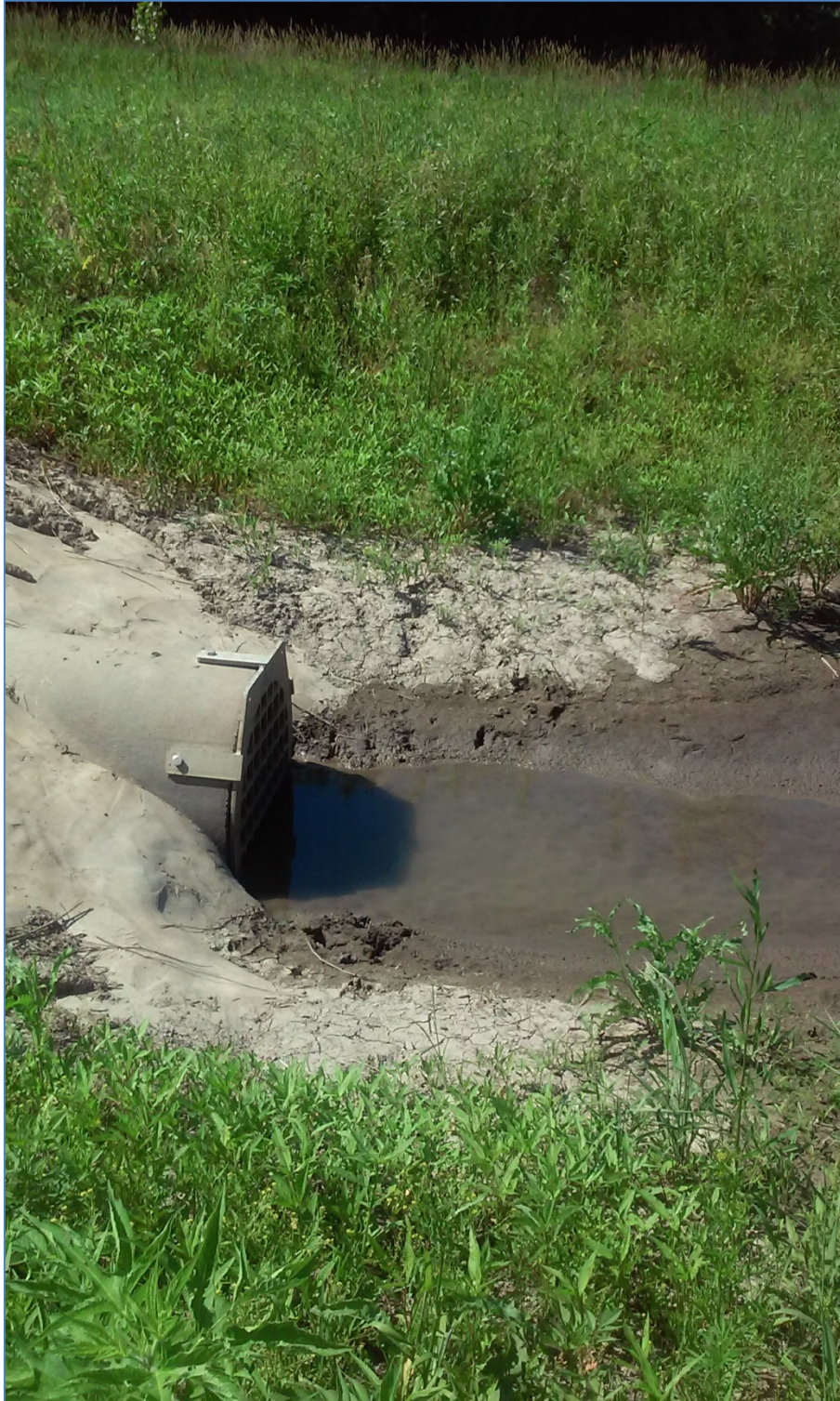
Photo #16 – Stoplog D, downstream gate, some erosion on either side.
