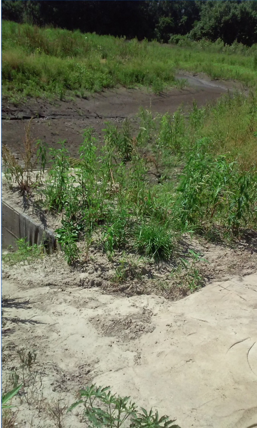
Photo #9 – Stoplog C, upstream gate. Sediment deposition and vegetation growth.
