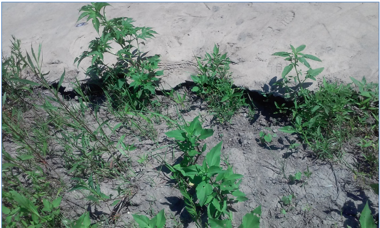
Photo #5 – Stoplog B, erosion at edge of riprap/concrete apron.
