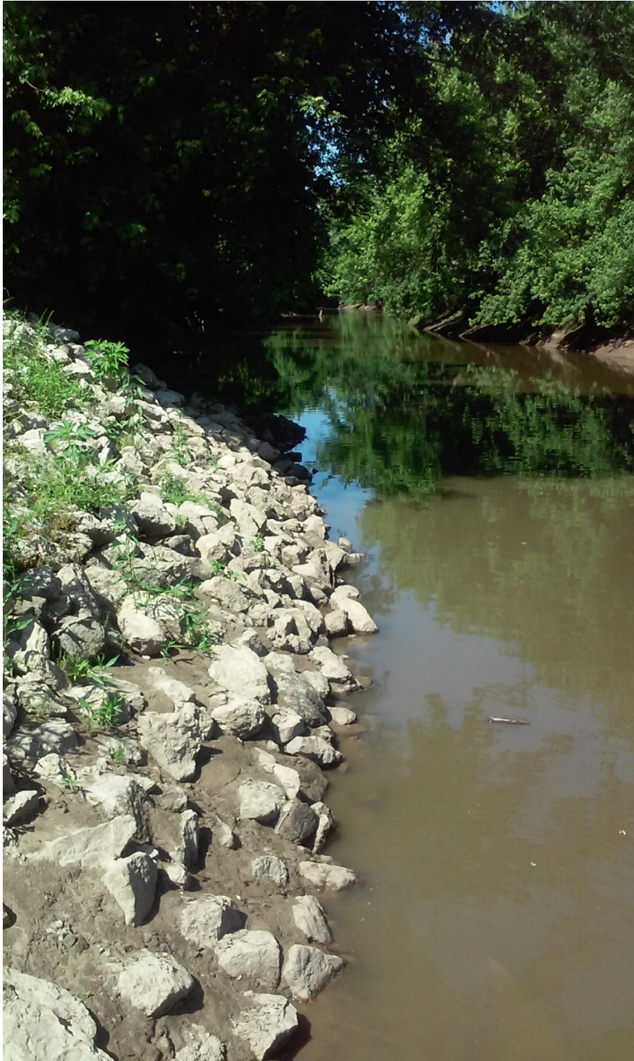
Photo #11 – Riprap downstream of Stoplog C. Some vegetation present.
