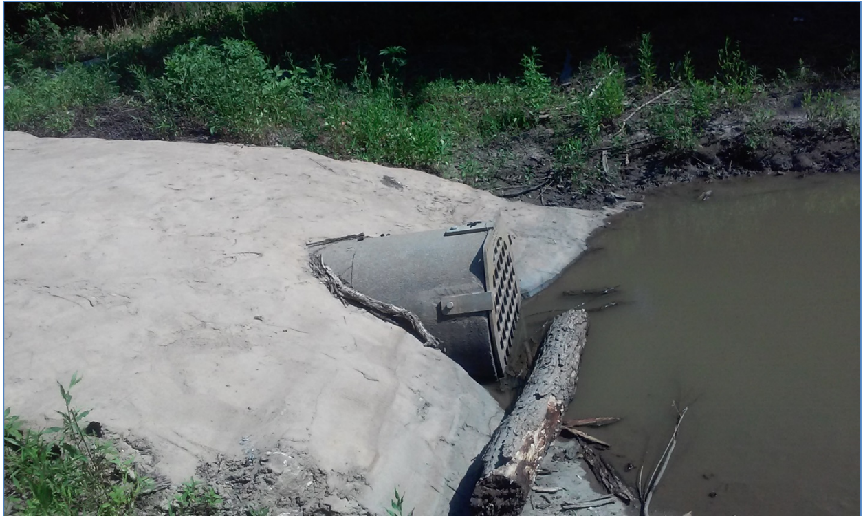
Photo #5 – Stoplog B, erosion at edge of riprap/concrete apron.
