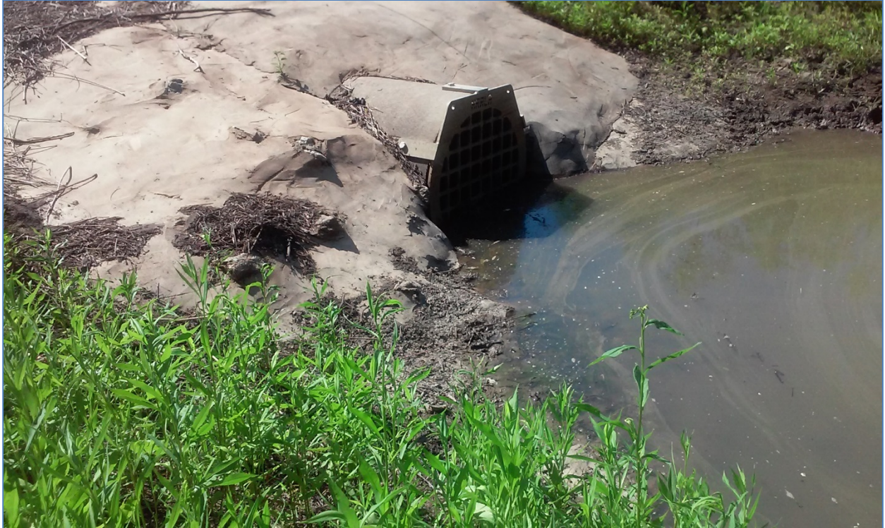
Photo #6 – Stoplog B, downstream gate.
