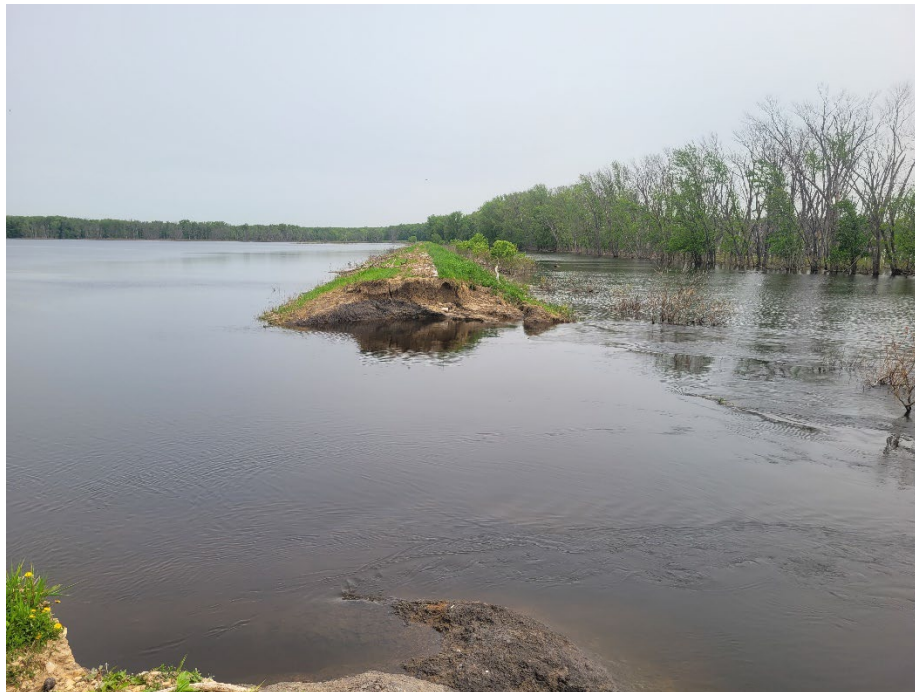
Figure C-4: Green Island Overtopping Breach Site Area
