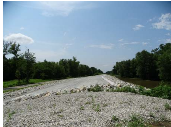
Photograph 81: Mississippi River Spillway (Mitvalsky, USACE 2016)
