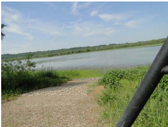
Photograph 12: Little Goose Pond Pump Pad (Mitvalsky, USACE 2013)
