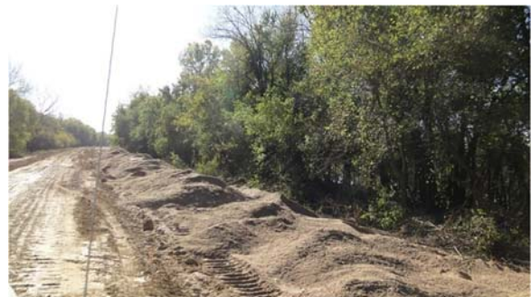
Photograph 64: Clay Cap Preparation (Mitvalsky, USACE 2011)
