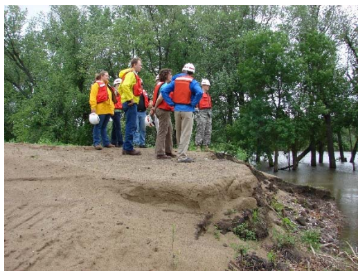
Photograph 185: 2008 Flood Damage Assessment (2008)
