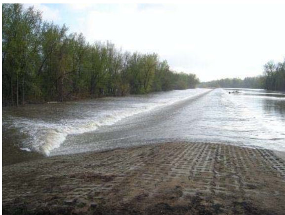
Photograph 85: Iowa River Spillway Overtopping (USACE 2008)
