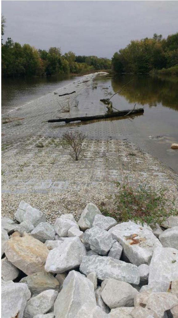
Photograph 93: New (Upstream) Iowa River Spillway Overtopping (Robbins, IADNR 10/3/2016)
