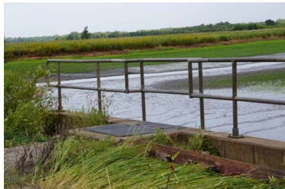
Photograph 22: Fox Pond at Water Control Structure (Mitvalsky, USACE 2016)
