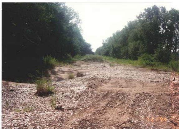
Photograph 55: Levee Pre-Project (USACE 1994)
