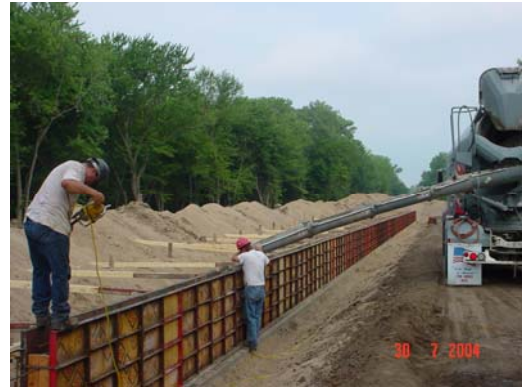
Photograph 193: Constructing the USFWS Spillway (2004)
