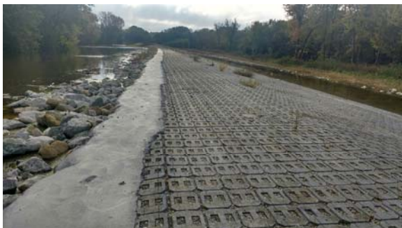
Photograph 94: Mississippi River Spillway (Robbins, IADNR 9/30/2016)
