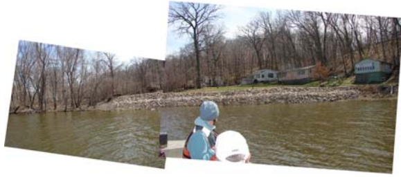
Photograph 147: Site 424 Erosion Protection (Mitvalsky, USACE 2009)
