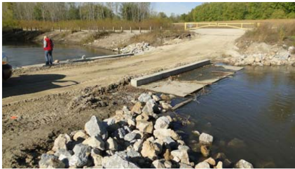
Photograph 78: Low Water Crossing at Inlet with Gate (Harper, USACE 2011)
