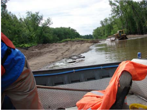
Photograph 60: Levee Repairs (Mitvalsky, USACE 2008)
