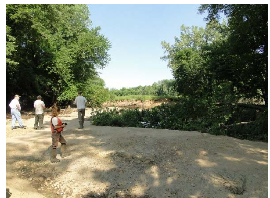
Photograph 165: 2014 Levee Breach Assessment (2014)
