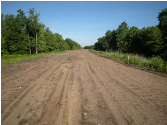
Photograph 61: Top of Levee before seeding (Mitvalsky, USACE 2012)
