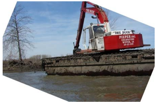
Photograph 49: Floating Excavator for Small Channel Cuts (Mitvalsky, USACE 2009)
