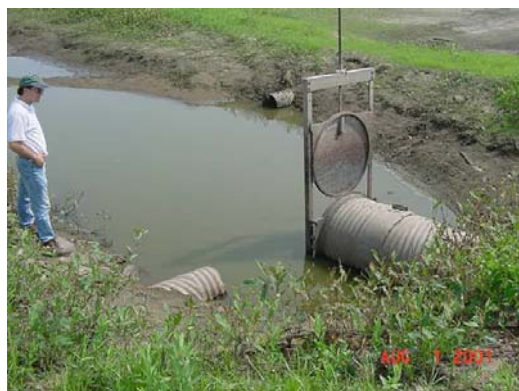
Photograph 198: Hydraulic Engineer Review of Water Control Structures (2001)
