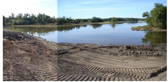
Photograph 123: Blackhawk Chute Excavation (USACE 2007)
