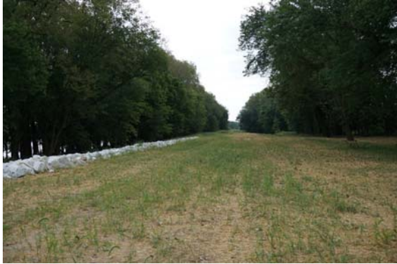
Photograph 71: Breach Repairs near Inlet (Mitvalsky, USACE 2016)
