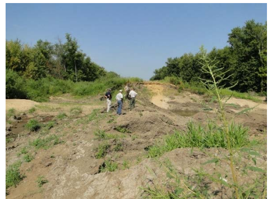
Photograph 170: Mississippi River Levee Breach near Outlet (USACE 2013)
