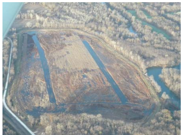
Photograph 40: IADNR MSU after final grading (IADNR 2012)
