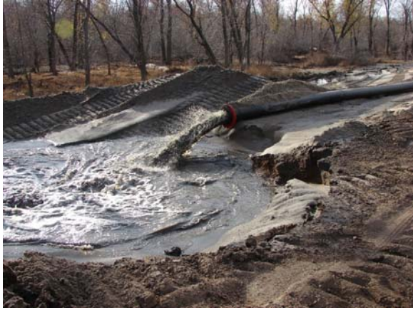
Photograph 59: Sand Embankment (USACE 2008)
