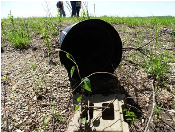
Photograph 36: IADNR MSU Water Control on Outside of MSU (Mitvalsky, USACE 2016)
