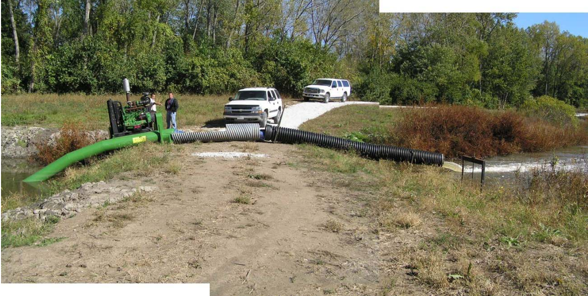
Photograph 16: Temporary Pump Filling MSU (Mitvalsky, USACE 2005)
