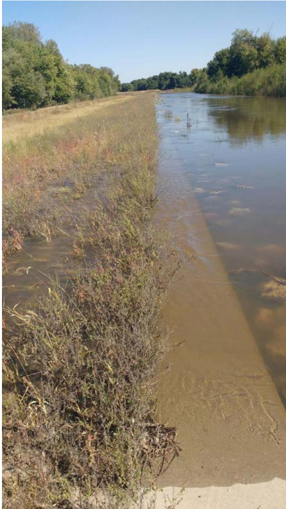
Photograph 89: Iowa River Spillway Starting to Overtop (Robbins, IADNR 9/29/2016)
