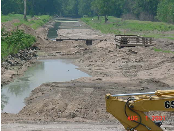
Photograph 4: Inlet Channel Preconstruction (USACE 2001)
