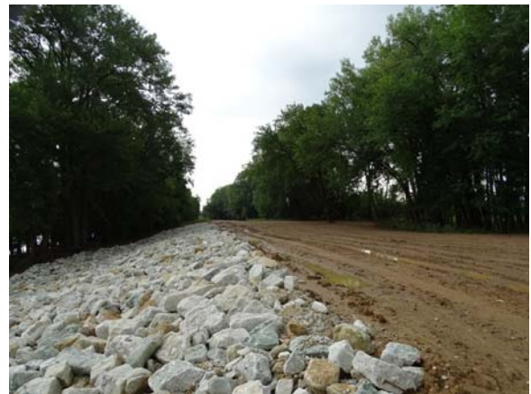
Photograph 70: Breach Repairs near Inlet (Mitvalsky, USACE 2016)
