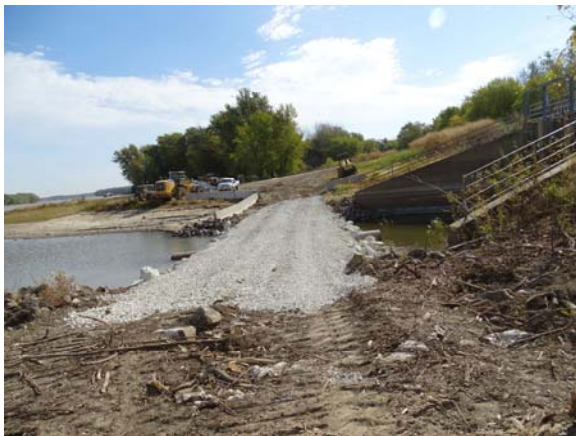
Photograph 79: Temporary Crossing near outlet (Mitvalsky, USACE 2015)
