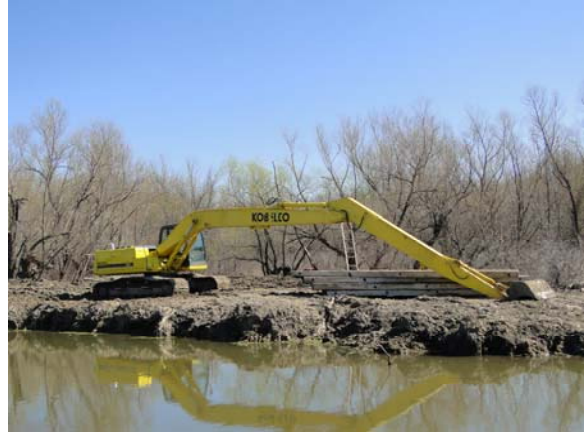
Photograph 111: Goose Pond Berm Shaping to Control Top Height (Mitvalsky, USACE 2011)
