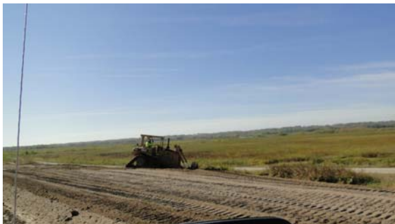
Photograph 67: Smoothing Out Side Slopes after Clay Cap in Place (Mitvalsky, USACE 2011)
