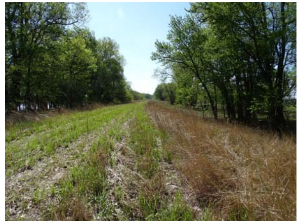
Photograph 69: Restored Levee (Mitvalsky, USACE 2016)
