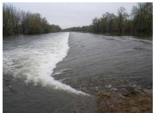
Photograph 88: Iowa River Spillway Overtopping (Robbins, IADNR 2011)
