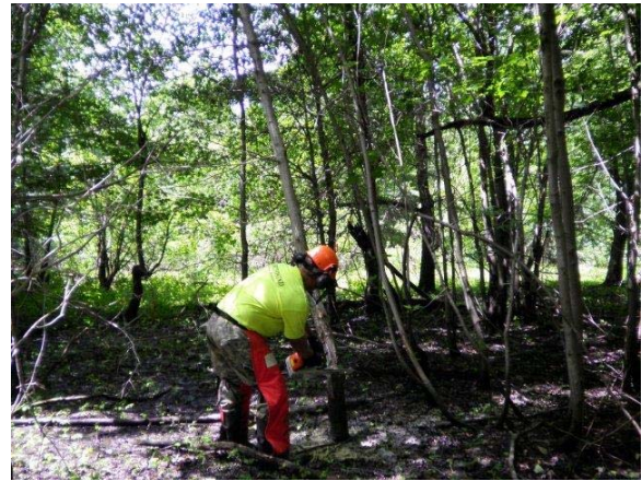
Photograph 134: Selective Tree Clearing (Lundh, USACE 2012)
