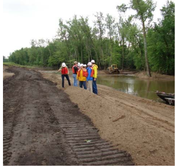
Photograph 62: Clay Cap preparation (USACE 2008)
