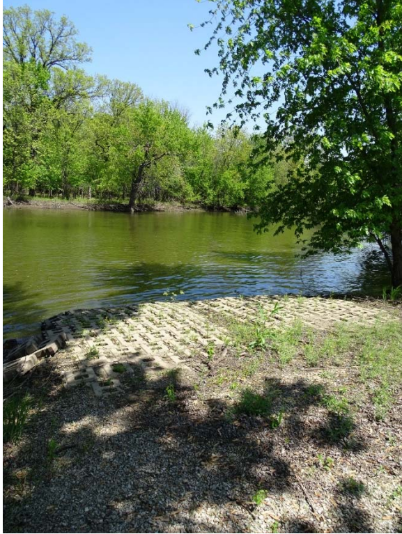
Photograph 46: IADNR MSU Pump Pad Leading into Burris Ditch (Mitvalsky, USACE 2016)
