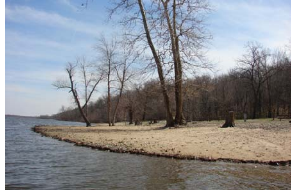
Photograph 144: Site 98 & 98 Riprap and Sand Protection (Mitvalsky, USACE 2009)
