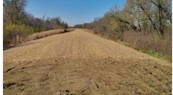
Photograph 68: Levee Repairs Post Seeding (Robbins, IADNR 2016)
