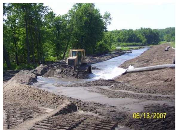
Photograph 58: Sand Embankment (USACE 2007)
