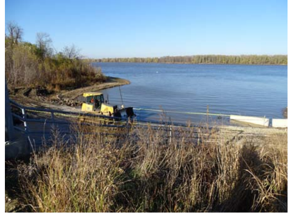
Photograph 80: Temporary Crossing near Outlet (Mitvalsky, USACE 2015)
