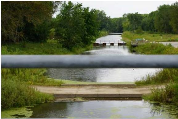
Photograph 5: Inlet Channel Excavation and Sidecast Material (Mitvalsky, USACE 2016)
