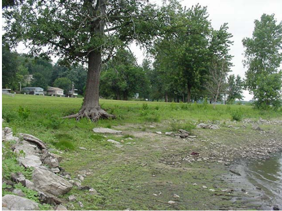
Photograph 141: Pre-Project Erosion Site 446 (Mitvalsky, USACE 2001)
