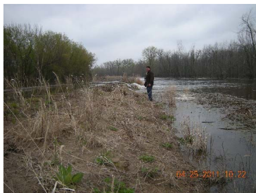
Photograph 172: 2011 Flood Damage Assessment (2011)
