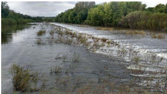
Photograph 90: Iowa River Spillway Overtopping (Robbins, IADNR 9/30/2016)
