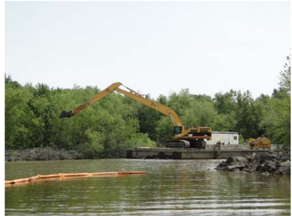
Photograph 105: Upper Goose Pond Cut (Mitvalsky, USACE 2010)
