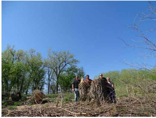
Photograph 160: Tree Clearing for Breach Repairs (2016)
