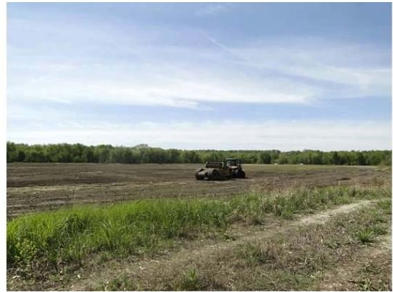
Photograph 39: IADNR MSU Final Grading (Mitvalsky, USACE 2012)
