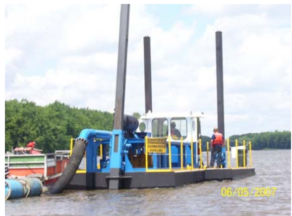
Photograph 57: Dredge for Levee Sand (USACE 2007)
