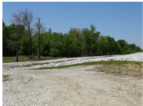
Photograph 82: Mississippi River Spillway Access Road around Structure (Mitvalsky, USACE 2016)
