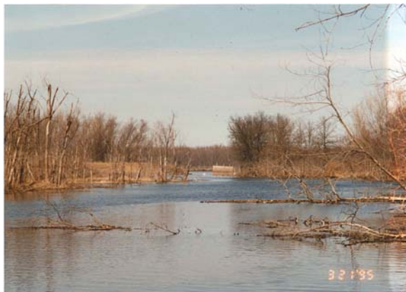
Photograph 73: Outlet Structure Being Constructed and Adjacent Levee Pre-Project (USACE 1995)
