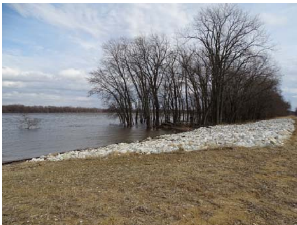
Photograph 72: Riprap Providing Flood Protection (Mitvalsky, USACE 2017)
