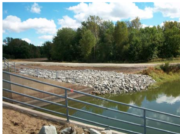
Photograph 76: Riprap at Outlet Structure (USACE 2009)
