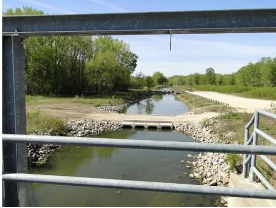
Photograph 77: Low Water Crossing at Inlet (Harper, USACE 2012)
