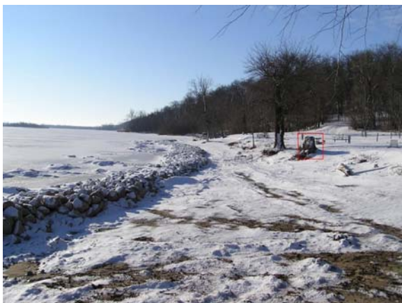
Photograph 143: Site 98 & 99 riprap only (Mitvalsky, USACE 2008)
