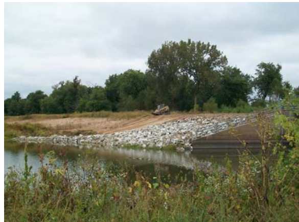
Photograph 75: Riprap at Outlet Structure (USACE 2009)
