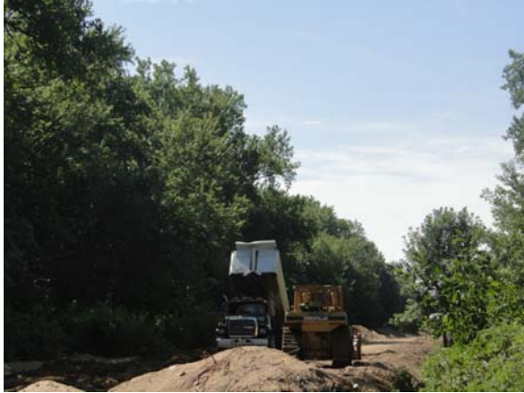
Photograph 65: Delivering Clay for Two Foot Clay Cap (Mitvalsky, USACE 2011)
