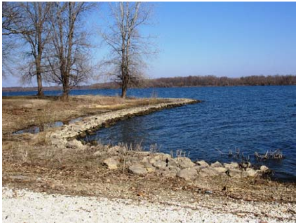
Photograph 142: Erosion Protection Site 446 (Robbins, IADNR 2017)
