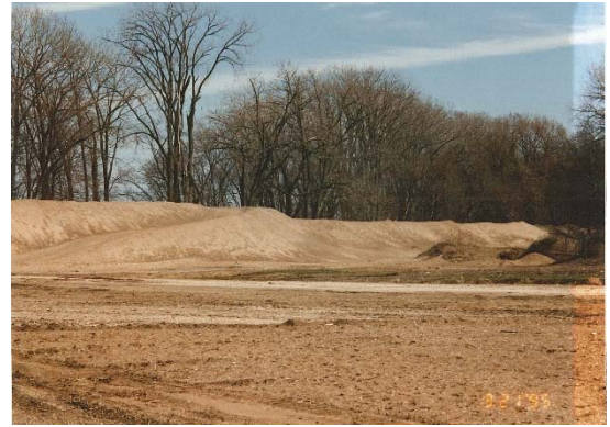
Photograph 204: 1993 Flood Damage Assessment (1995)
