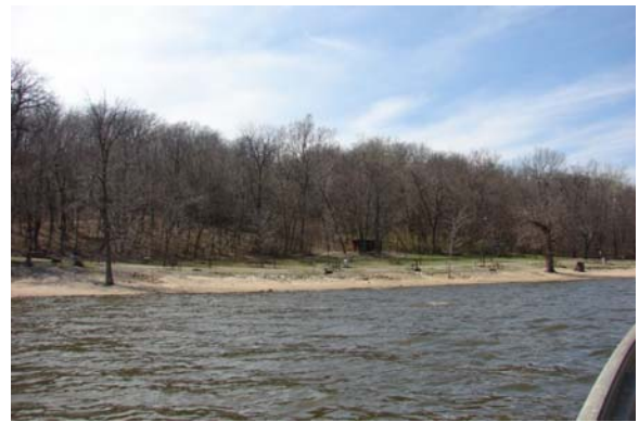
Photograph 145: Site 98 & 99 erosion protection (Mitvalsky, USACE 2009)
