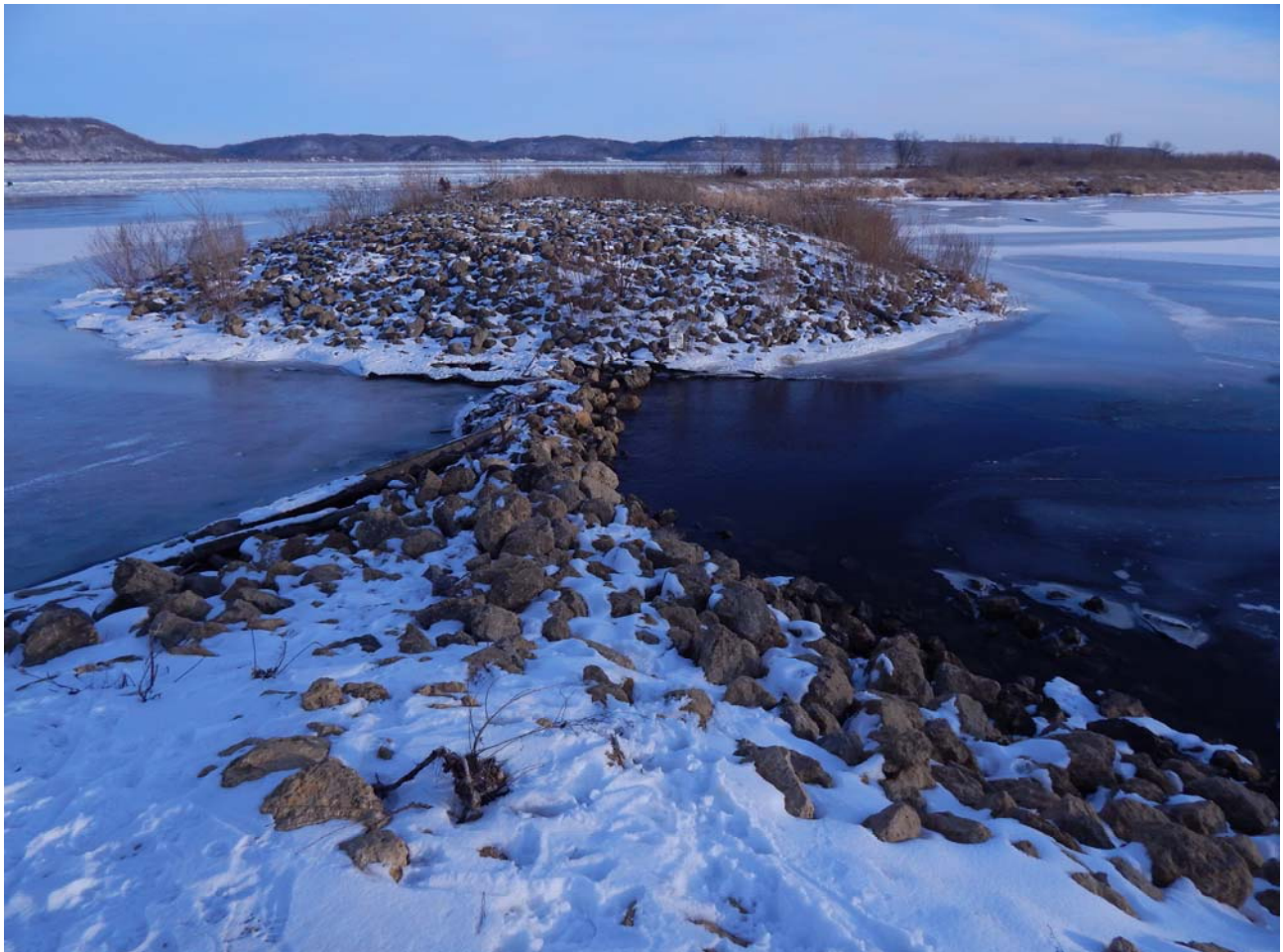
Rock-filled upper inlet of the Mud Lake portion of the Pool 11 Islands HREP (Courtesy of Scott Gritters, Iowa DNR).
