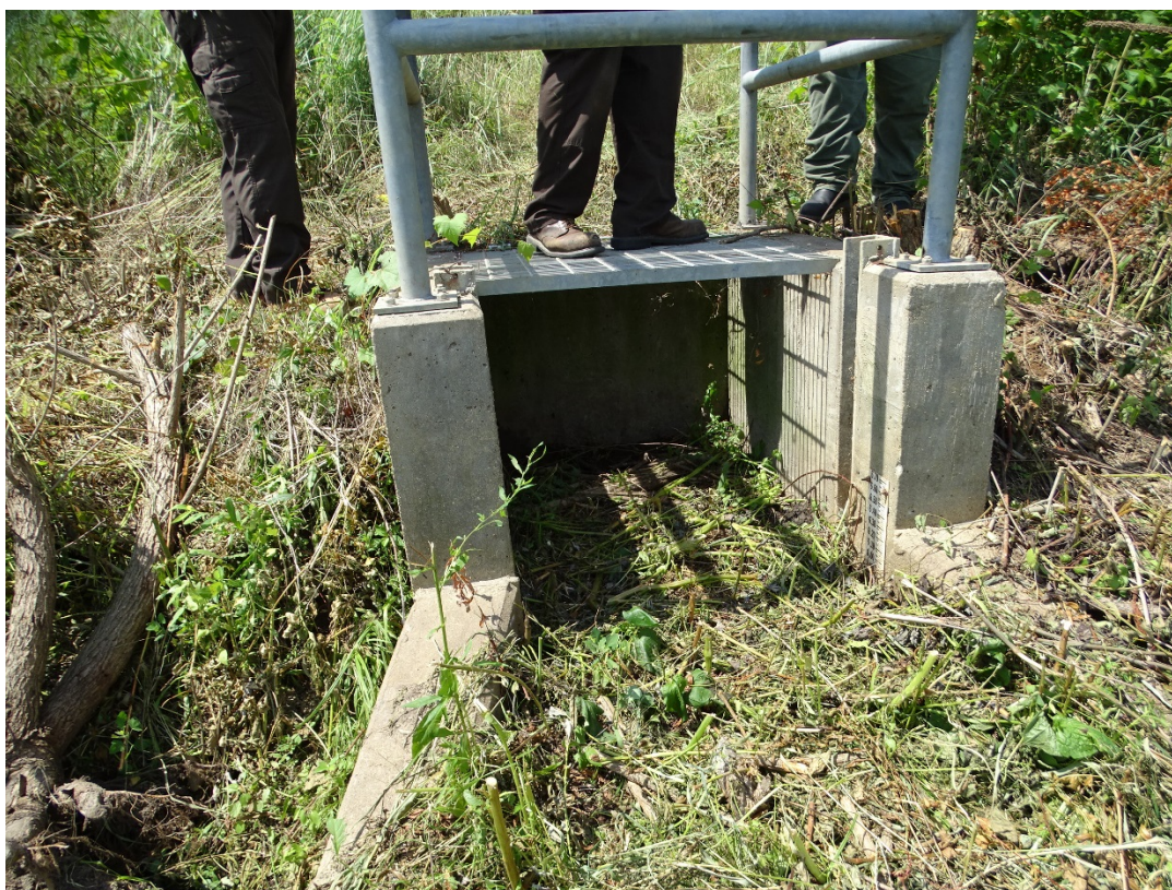
Photo 12: Stoplog structure
