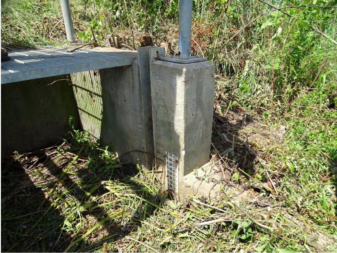
Photo 13: Stoplog structure and gage
