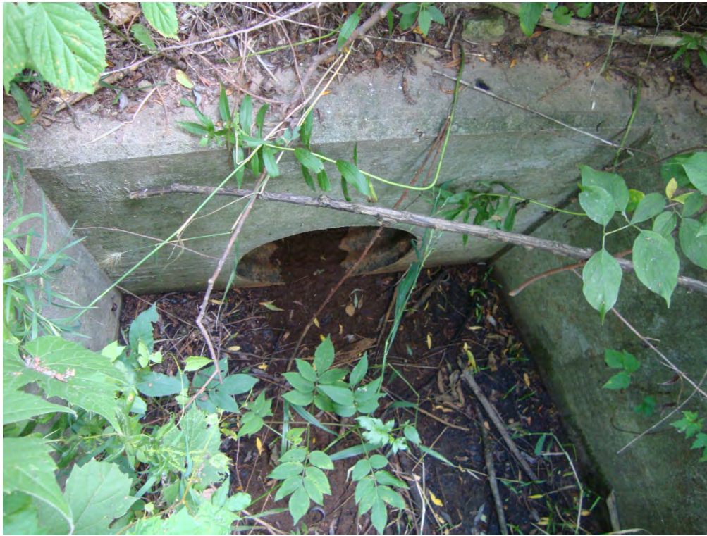
Photo 11: Stoplog structure outlet headwall.
