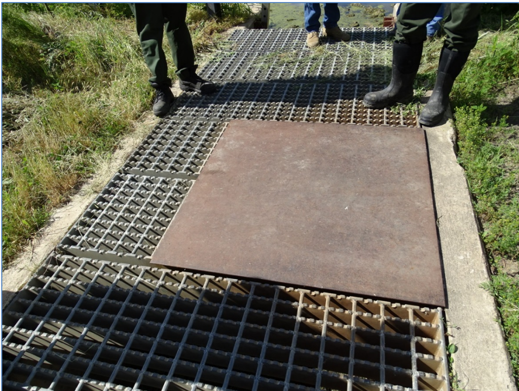
Photograph 12: Pump Station Outlet. Metal plate added to reduce water splashing out of structure
