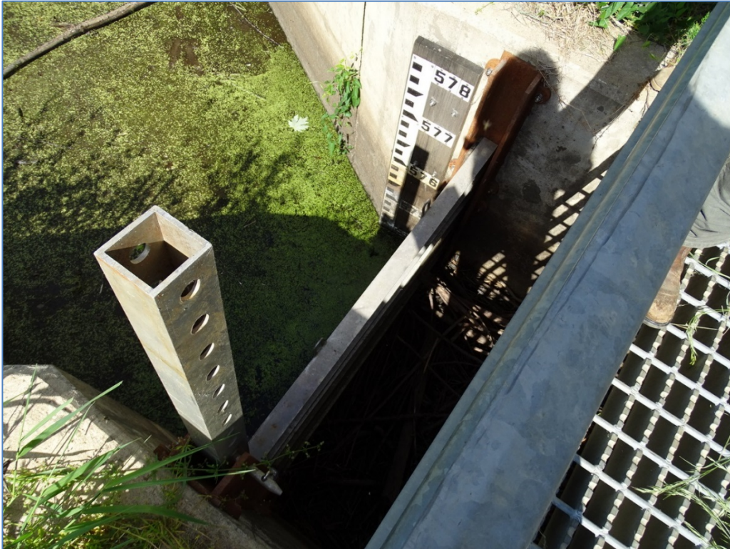
Photograph 11: Stoplog Structure Near Pump Station
