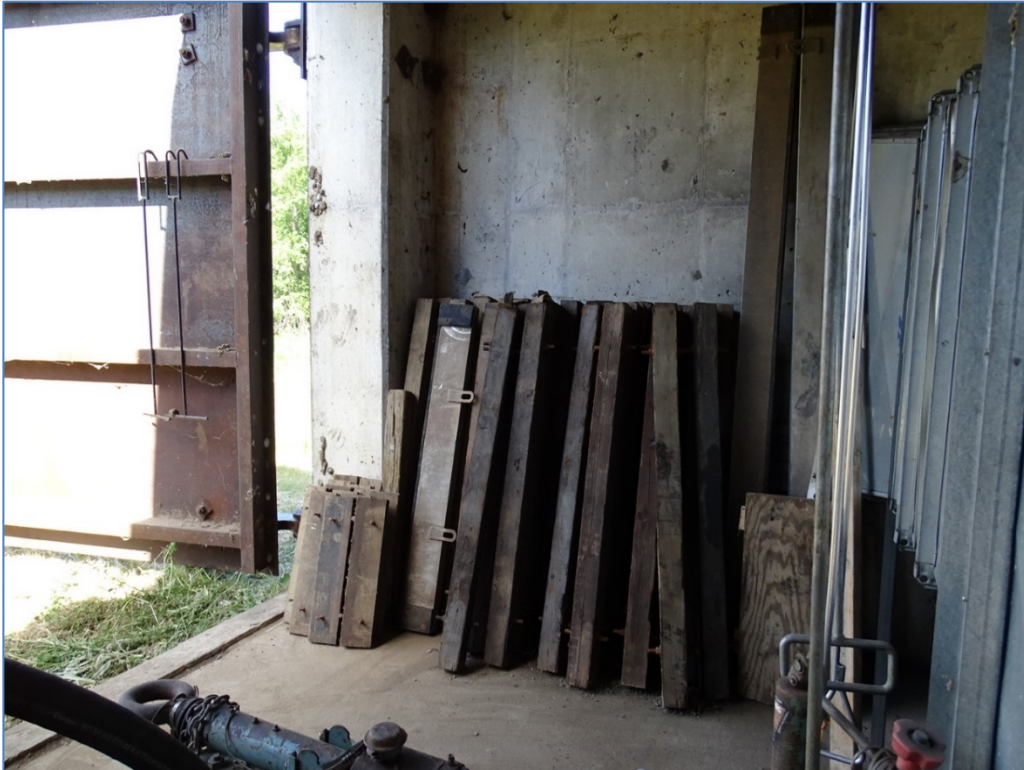
Photograph 9: Stoplogs for water control structures (stored in the pump house)
