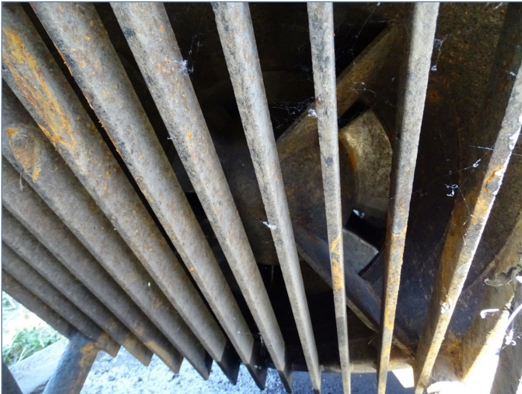
Photograph 10: Pump Intake (pump had been pulled and was being stored in the pump house).
