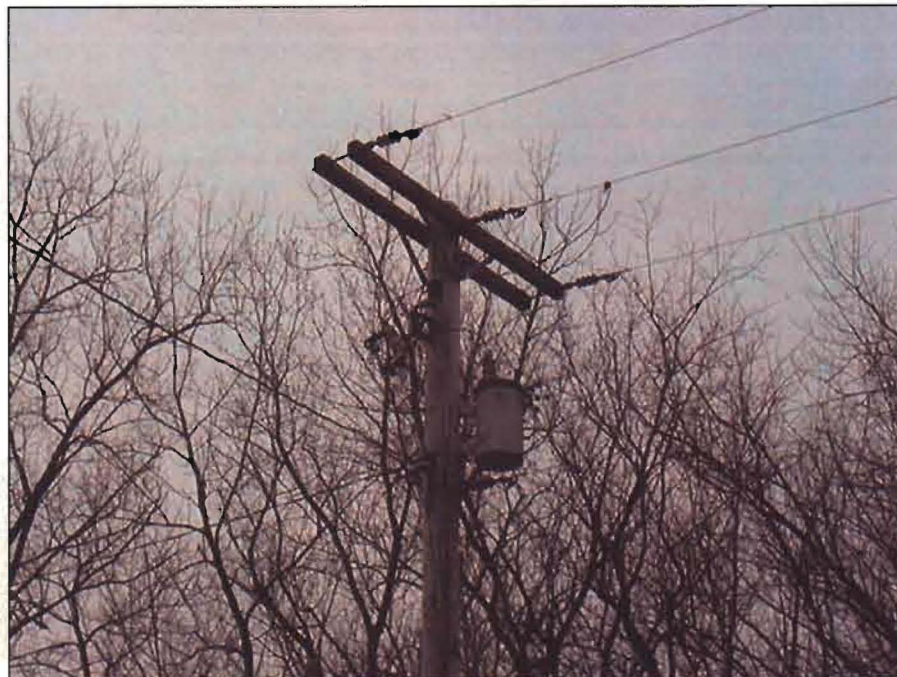
Photo D022. Single-phase 220 VAC Power Source for Public Use Area.
