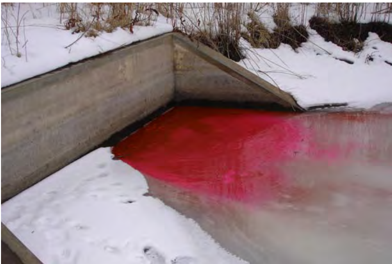
Figure 4. Dye entering Spring Lake at the water control structure.
