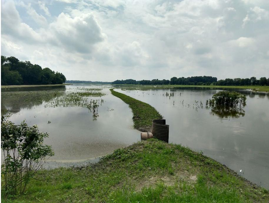
Figure 1. Existing CMP Water Control Structure and Berm
