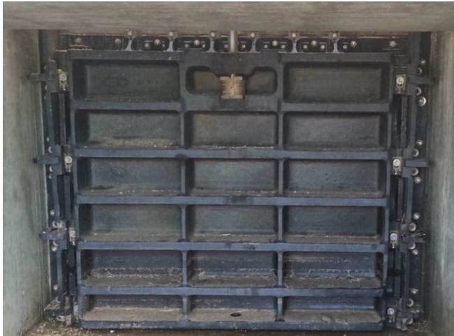
Figure 6. Cast Iron Sluice Gate
