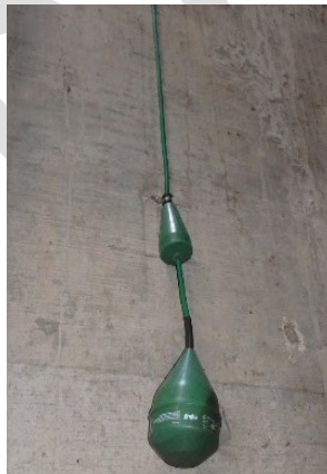
Figure 5. Low Water Cutoff Float Switch
