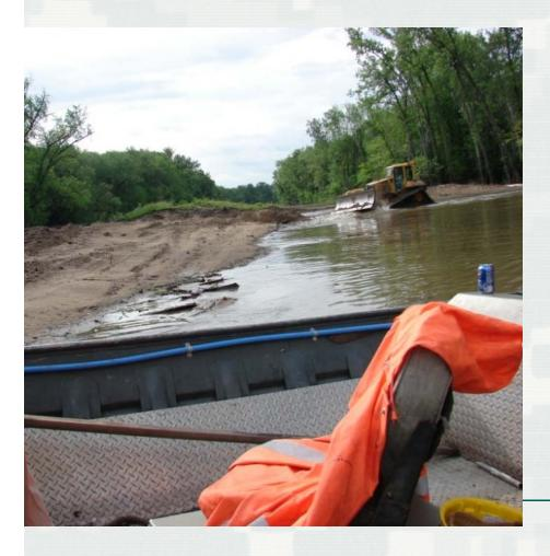
Remove sediment which has entered system through previous breaches
