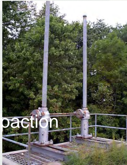
Sluice Gates
