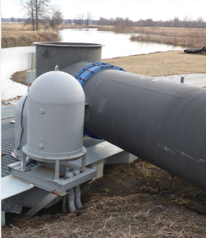
One Unique Method of Flood Proofing – Steel Bell Installed Over the Top of Electrical Equipment to Provide Air Pocket
