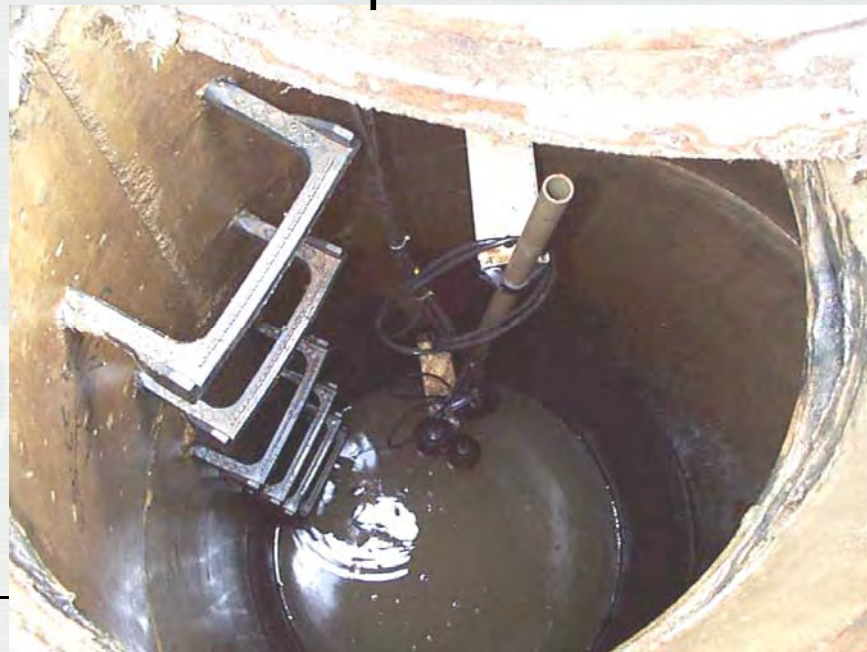
Float Well w/ Encapsulated Floats
