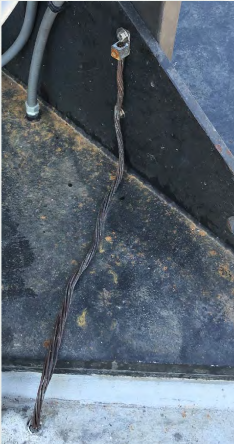
Equipment Grounding Wire
