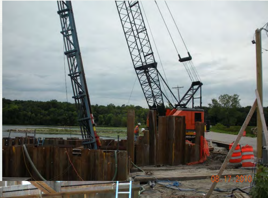
Battered Pile Installation
