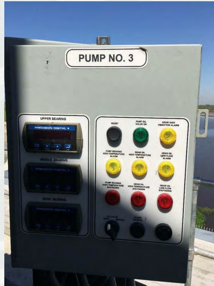
Outdoor Pump Alarm Panel
