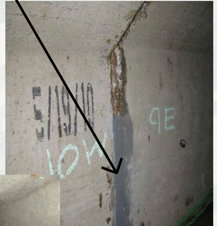
Conduit Joint Repair
