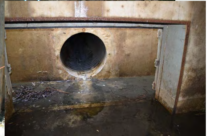
Conduit w/ Spiral Sleeve
