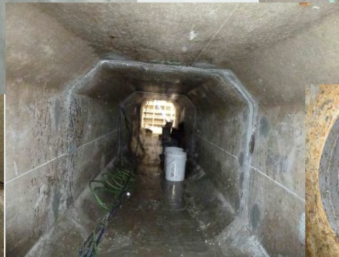
Conduit Joint Repair
