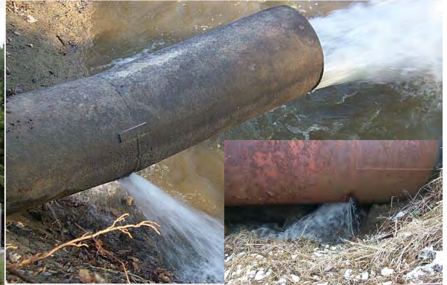
Discharge Pipe w/ Erosion
