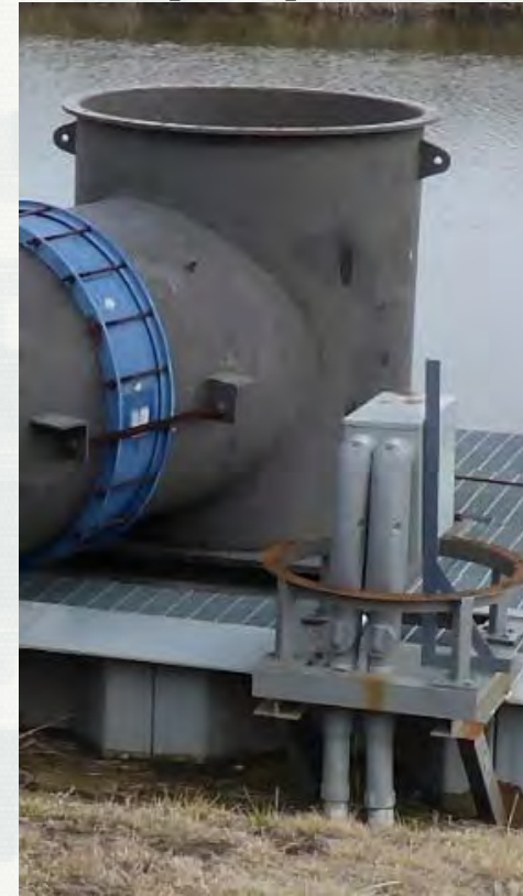
Steel Bell Removed Reveals The Pump Electrical Equipment
