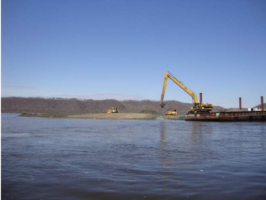
Employees of Newt Marine Services of Dubuque use heavy equipment recently to build islands in Harpers Slough in the lower part of pool 9 of the Mississippi River. The project, which began in April, consists primarily of backwater dredging and the construction of seven islands encompassing more than 100 acres. U.S. Fish and Wildlife Service photo
