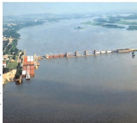
Locks and dams such as this one near Bellevue, Iowa establish boundaries of the navigation pools.
