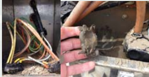
Water intrusion on junction box and pumps 17-Sep-15
