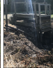
Water Control Structures
