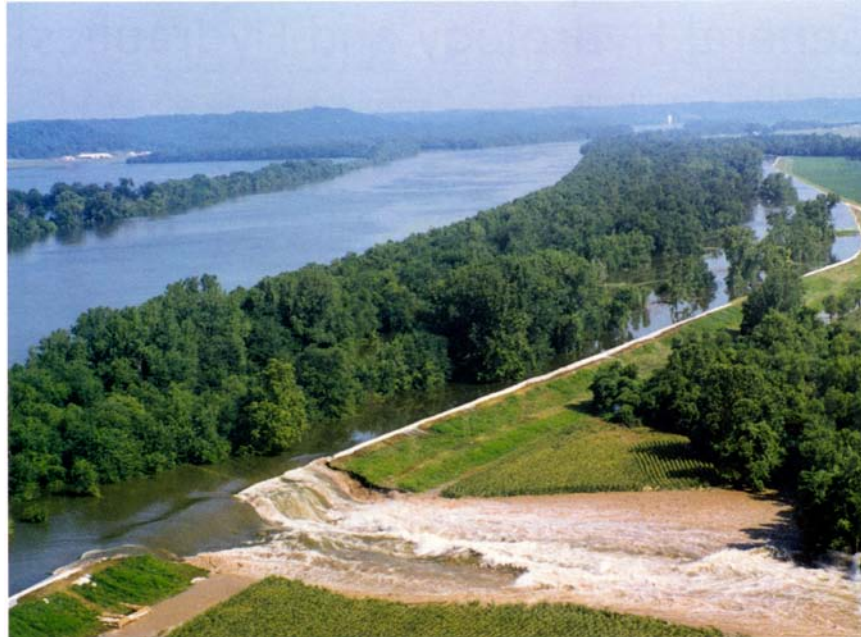
Figure 1. Levee Breach (North Central Division, 1994)
