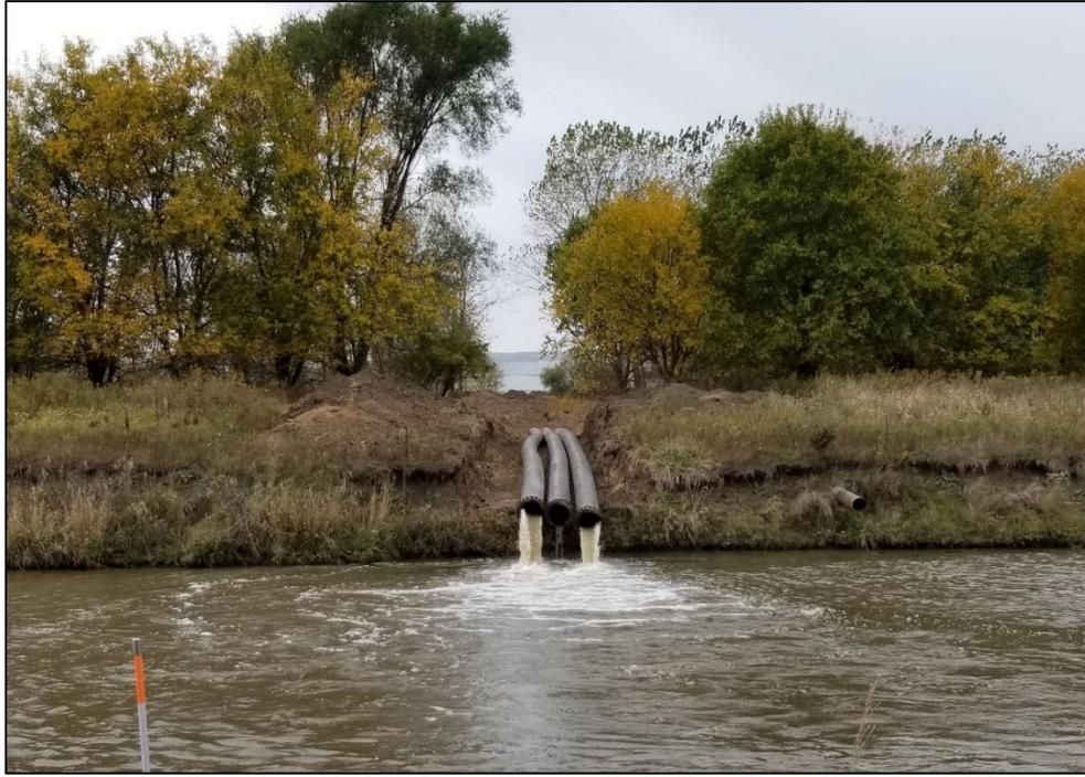
**Photograph 3.** Example of the Return Water Method to Be Used at Buffalo DMMP Site 5, Using Three 20-inch Diameter Pipes Temporarily Placed in an Excavated Gravity-Flow Ditch
