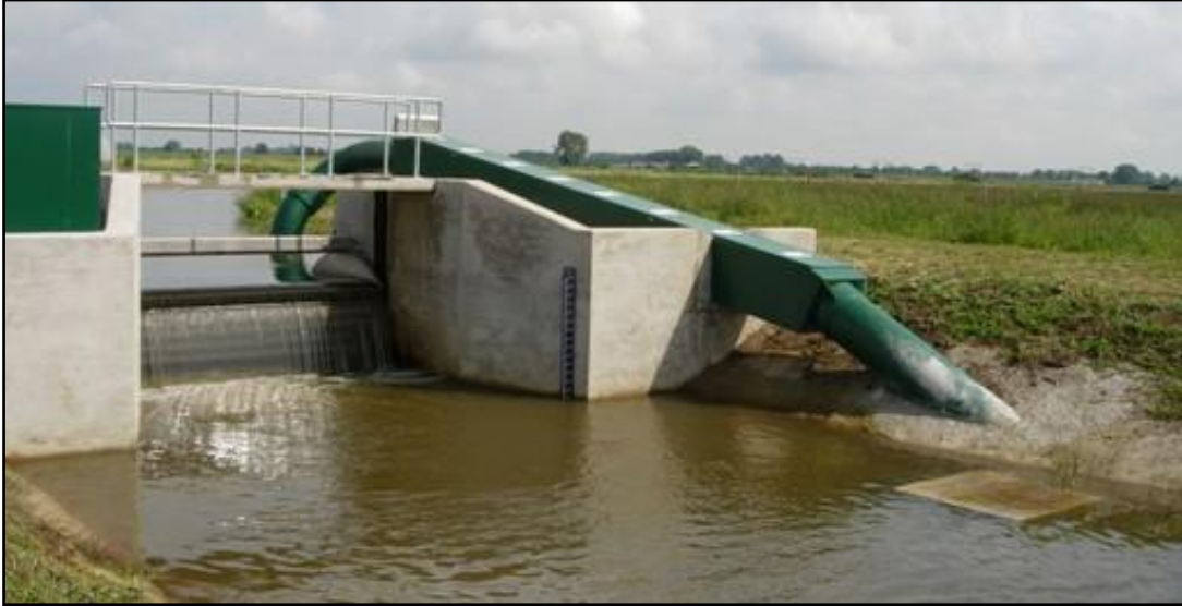
Photograph 8. Fish Siphon (FishFlow Innovations)
