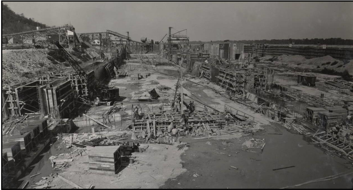
Photograph 3. Main Lock Construction, October 1934
