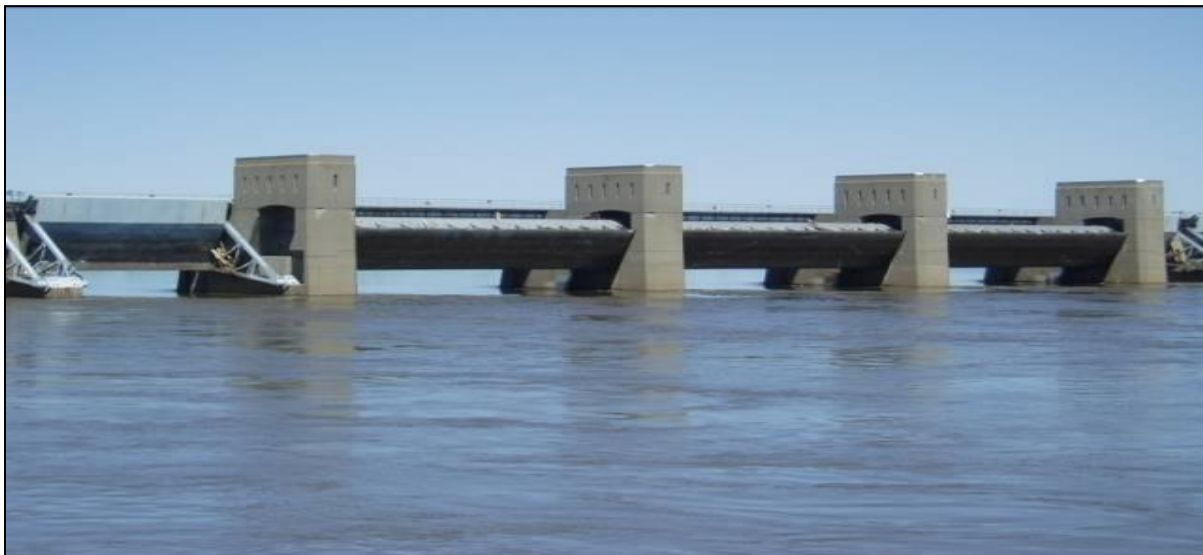
Photograph 6. Roller Gates at Lock and Dam 22 During Open River Conditions
