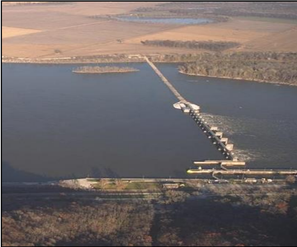
Photograph 5. Lock and Dam 22 Looking East Toward Illinois
