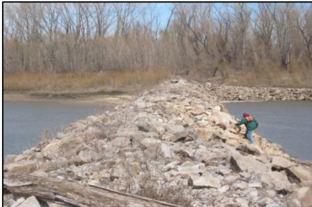
A prototypical stone dike constructed within the middle Mississippi River
