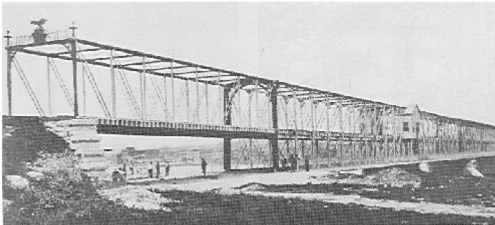
In 1872, another bridge was built to replace the wooden one. However, the location was changed. This bridge was built on the same site as the present day Government Bridge. It consisted of a single rail line above a wagon path. The train track was designed to be on top because the smoke and noise frightened horses when trains ran under them.
