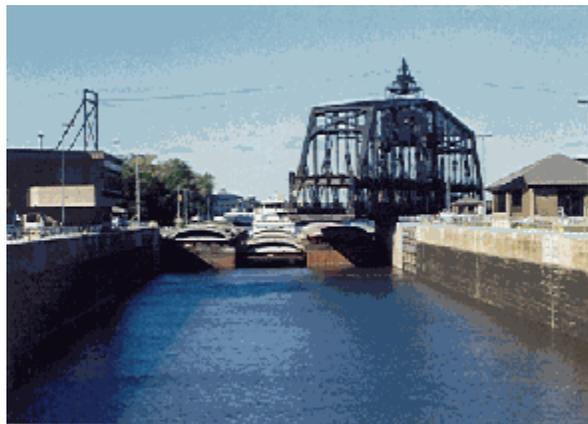
Bridge personnel are on duty 24 hours a day. They have to be able to open the bridge anytime a large boat like a towboat with barges needs to go through. The bridge operator controls the swing span from the house located on top. A "ground person" used to be needed to make sure all traffic was off the bridge before it was turned. However, today the bridge has been equipped with numerous cameras that the operator can monitor and be sure that the bridge is all clear before moving.
