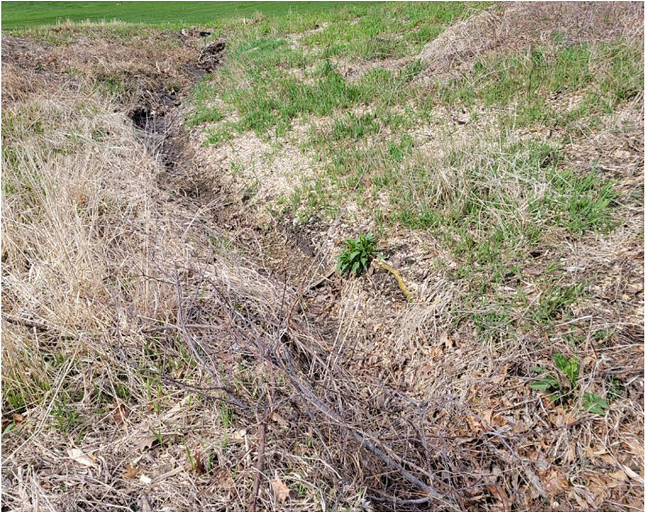
D-3 is a drainage swale fed by a tile from the uplands.
