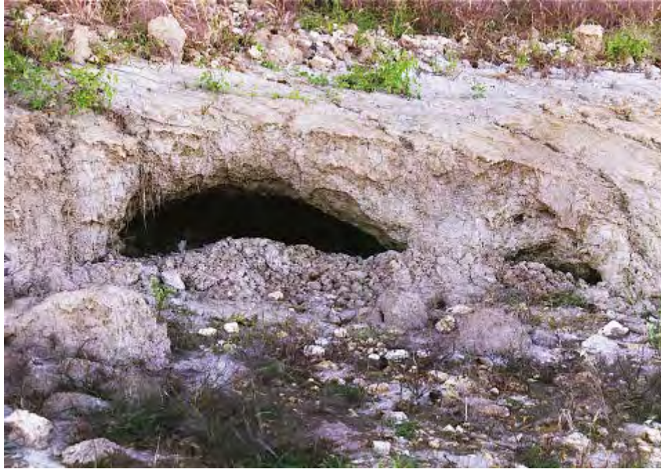
Photo 7-116 Piping features of Site 41 midpoint
