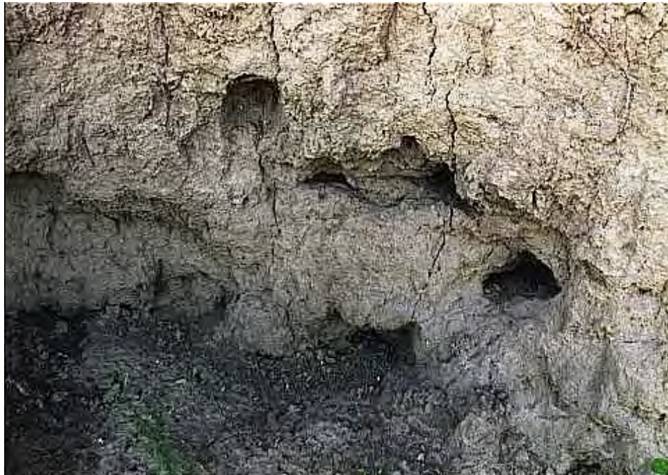
Photo 7-64 Piping features and vertical cracks seen at Site 28 midpoint
