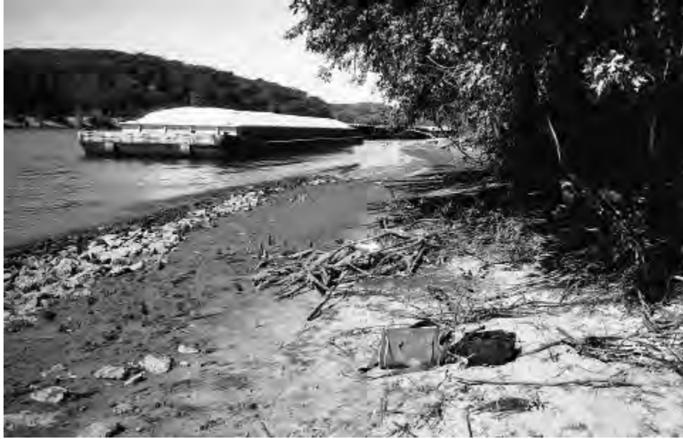
Photo 7-7 Severe bank erosion at barge mooring area observed at Site 15, RM 576.0
