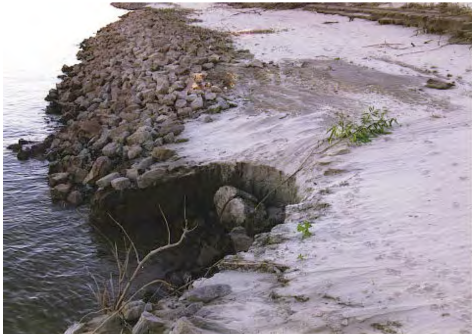
Photo 7-118 A close-up view of revetment failure at Site 42 midpoint
