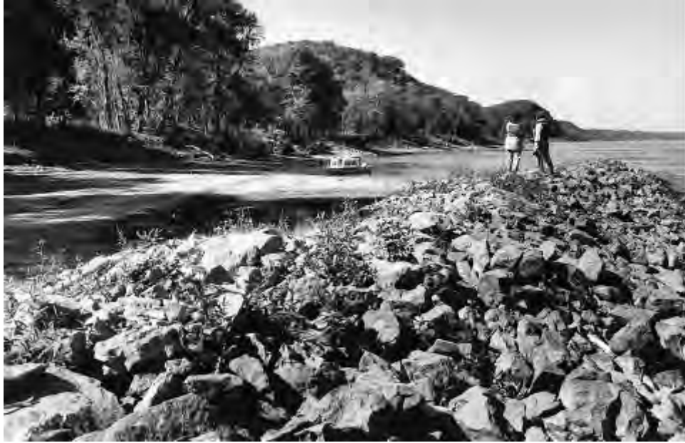
Photo 7-9 Observation Site, RM 134.1 -- looking north upstream -- (this photo shows study team members standing on CCC-placed riprap (ca. 1930s) About 150 ft of bank erosion has occurred westward to the left since riprap placement)
