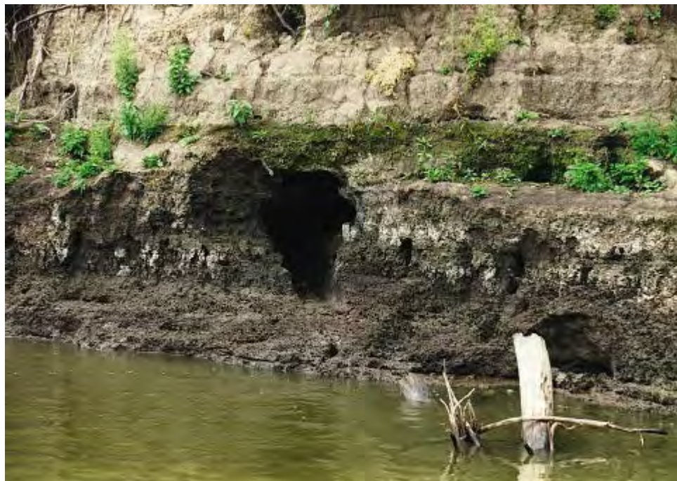
Photo 7-73 Close-up of piping features - Observation Site at RM 322.9 RDB
