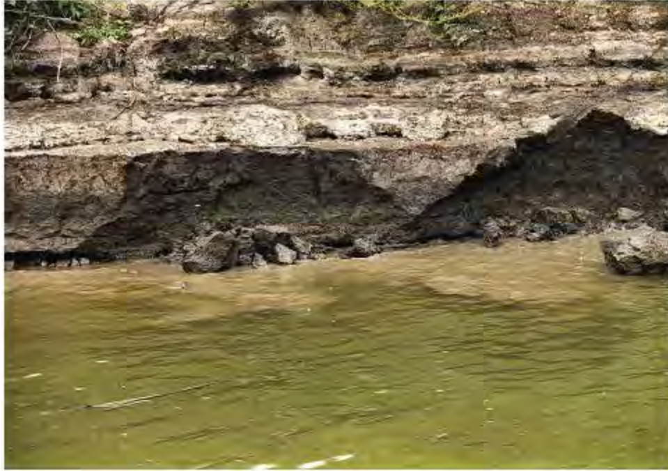
Photo 7-76 Vertical failure of lower bank - Observation Site at RM 322.9 RDB
