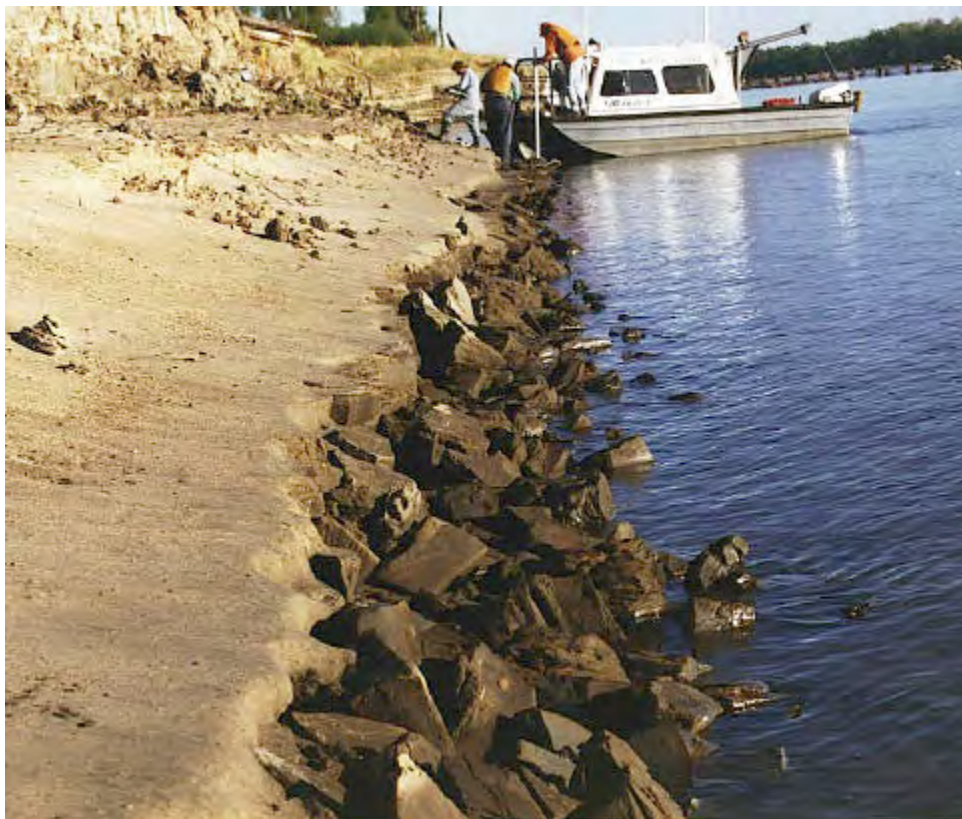
Photo 7-110 A close-up view of eroded bench at Site 39 midpoint
